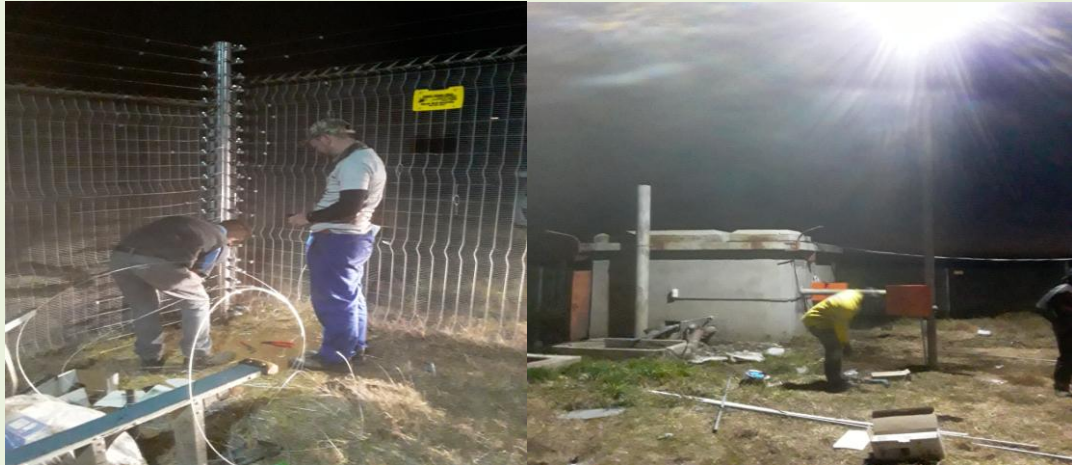
Installation of an electric fence at West Pump Station & Installation of electronic security systems at West Pump Station
