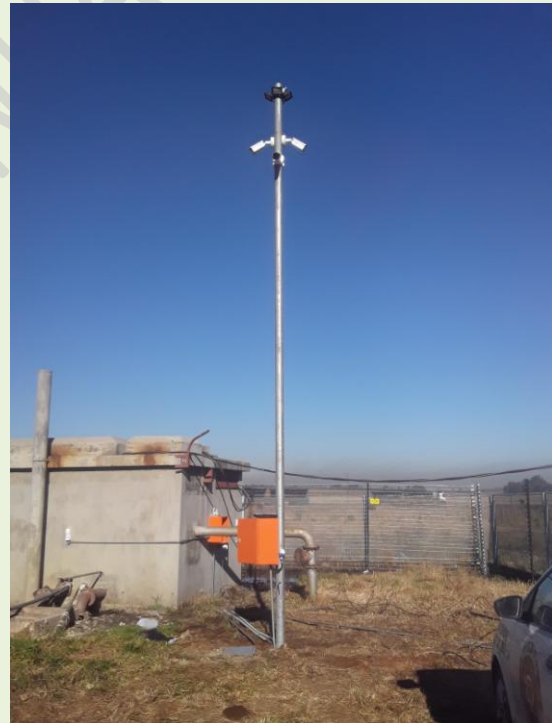
Installation of an electric fence at West Pump Station & Installation of electronic security systems at West Pump Station
