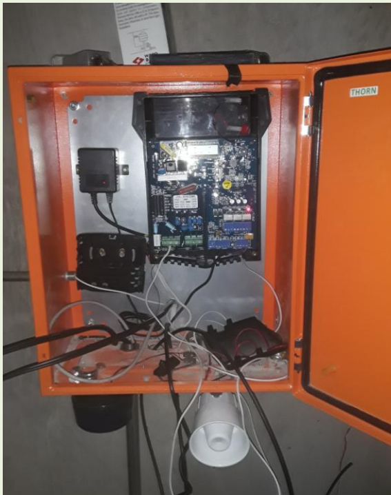
Installation of an electric fence at West Pump Station & Installation of electronic security systems at West Pump Station
